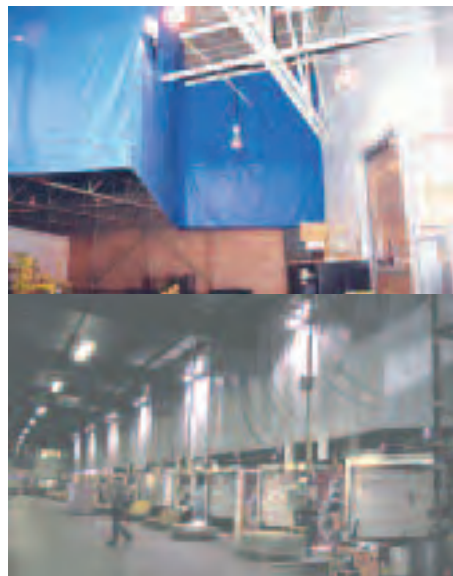
These suspended hoods help contain and control truck exhaust fumes.
