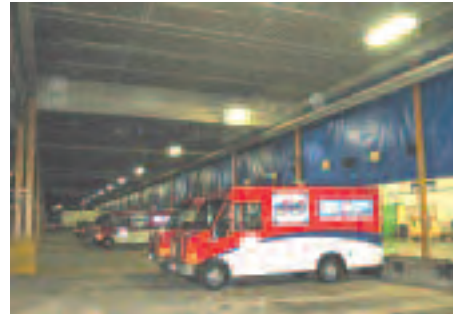
These suspended hoods help contain and control truck exhaust fumes.
